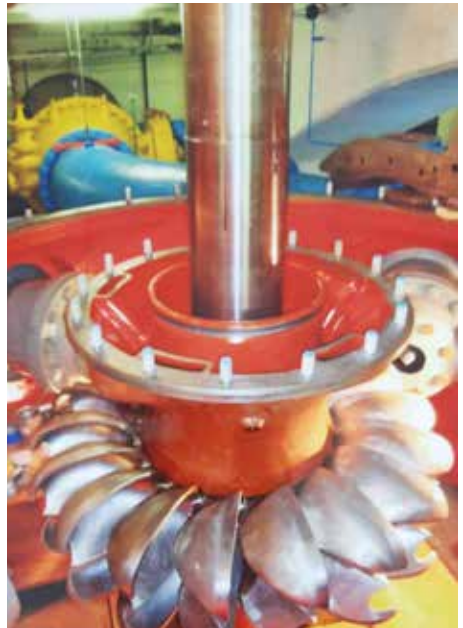
Turbinenrad in Revision.
